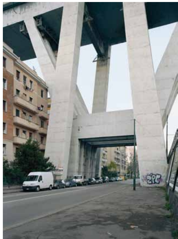
Abb. 1: Riccardo Morandi, Autobahnbrücke, 1960–1967, Genua © Werner Feiersinger
